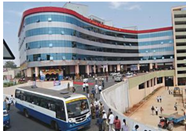
Figure 9 Traffic and Transport Management Centre in Bangalore (BMTc 2014)
