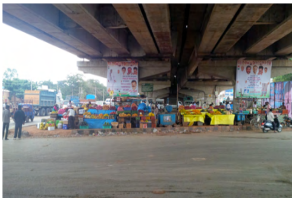
Figure 42 The grade-separated Chandapura Junction (EMBARQ India 2014)
