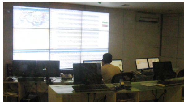
Figure 61 Janmarg BRTS Control Centre (EMBARQ India 2014)
