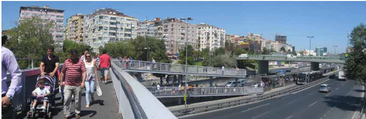
Elevated pedestrian bridges to Metrobus
